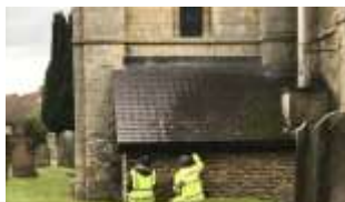
Stonework repairs being carried out at the Church.
